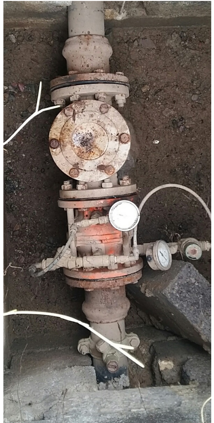
Old PRV due for replacement at Clough, Longford
